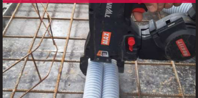
Electrical and plumbing piping
