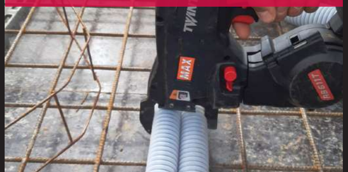
Electrical and plumbing piping
